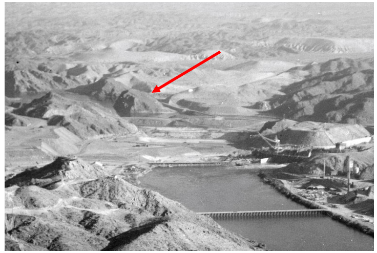
Aerial view from south of the construction of Davis Dam. Just above the coffer dam one can see the Bullshead Rock formation.
