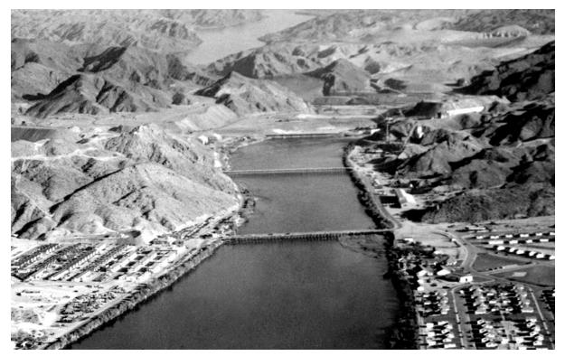
Looking north during construction of Davis Dam. Arizona is on the right side and Nevada to the left. In the foreground are the temporary construction bridges. Demolished after the completion of the dam, there would not be another bridge built until 1987 when Don Laughlin built a public bridge downstream near his Riverside Casino.
